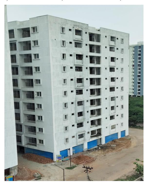
**Block D3: Terrace** Floor level slab Concrete casting 100% completed. External Plastering work overall 95% completed. 1<sup>st</sup> Coat of Primer 75% completed.
