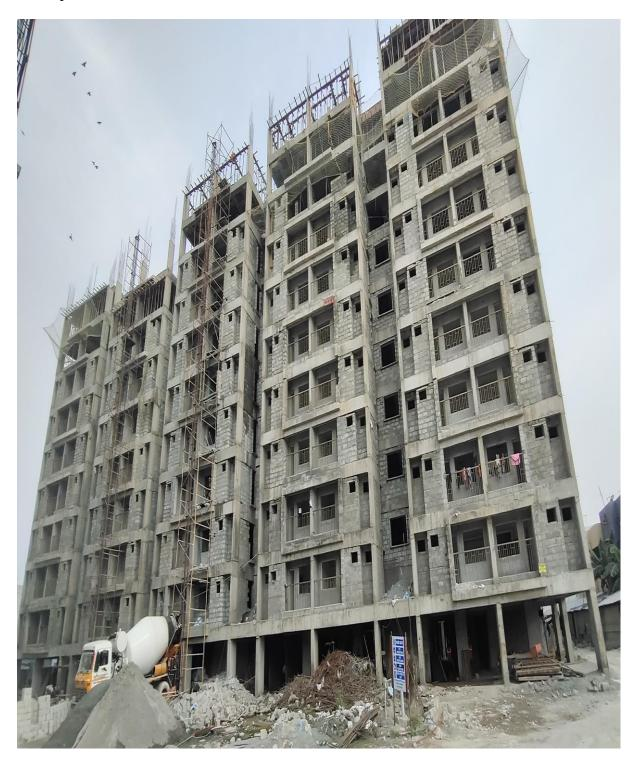
**Block A2:** Tenth Floor level slab  $-1^{st}$  Half Concrete casting 100% completed.
