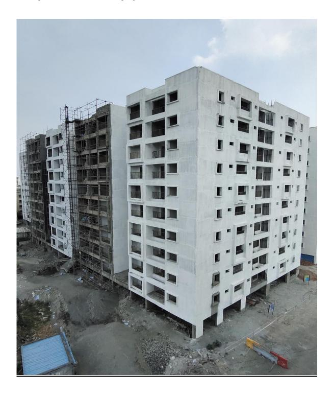
**Block D2:** Over Head Water Tank 100% completed. External Plastering work overall 95% completed. 1st Coat of Primer 85% completed. Installation of Lifts 50% completed.
