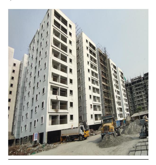
**Block D1: Terrace** Floor level slab Concrete casting 100% completed. External plastering overall 70% completed balance works on progress.
