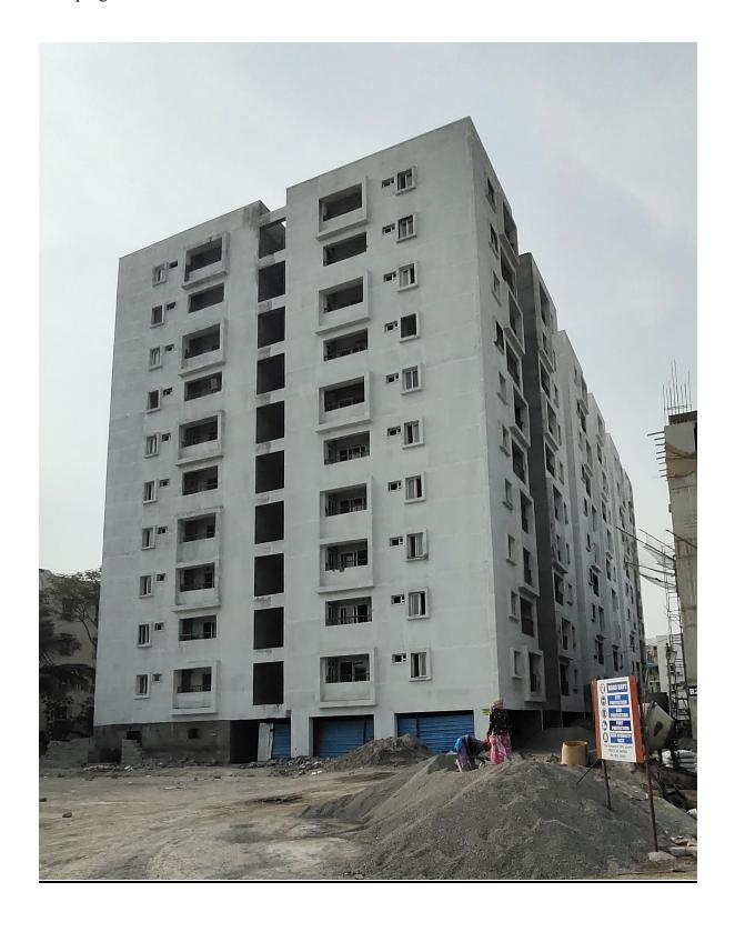
**Block B2:** Fourth Floor Level slab concrete casting 100% completed. Shuttering works for  $1^{st}$  half of Fifth floor level slab 50% completed.
